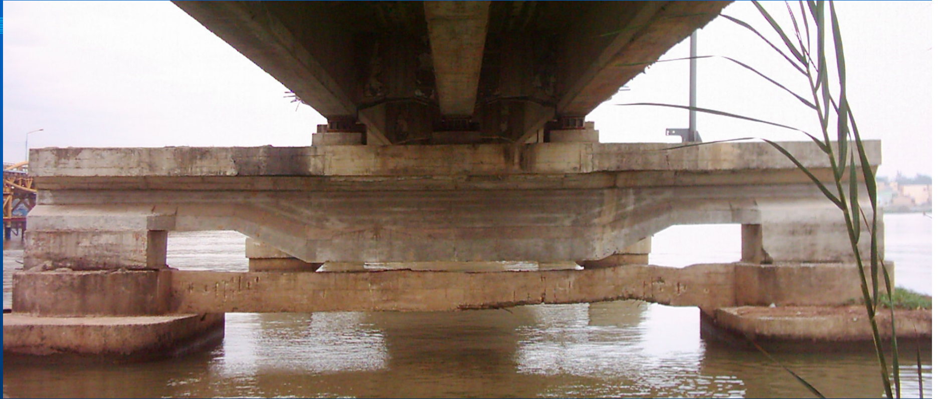
Picture 3: Head beam have been repaired by polymer mortar and additional bonding steel plates
