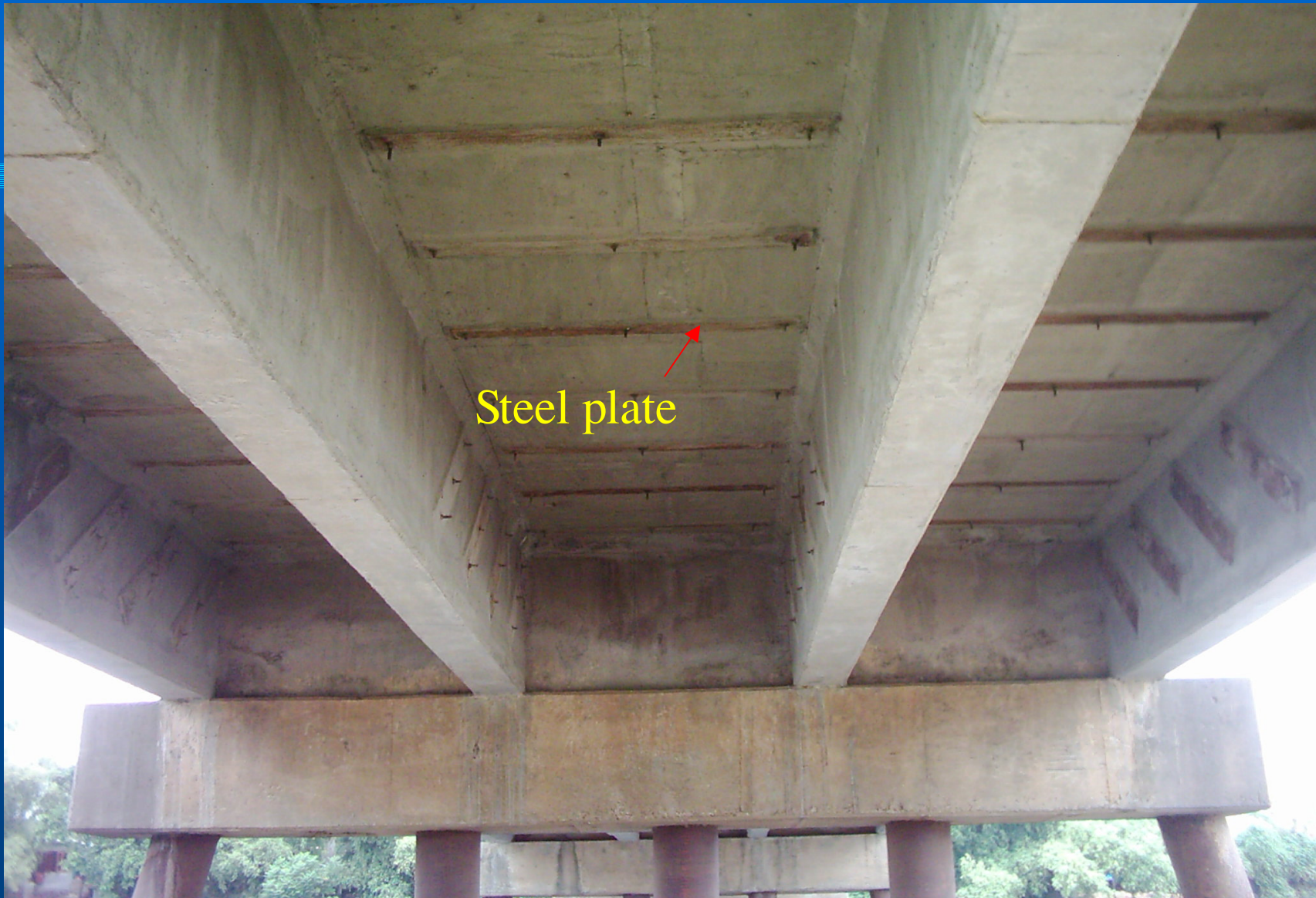
Picture9: Span structure of Ba – Ren bridge (8/2005)
