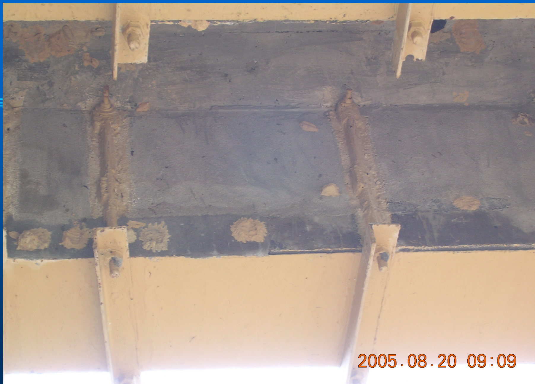
Picture 20: The steel plates at the bottom of beam
