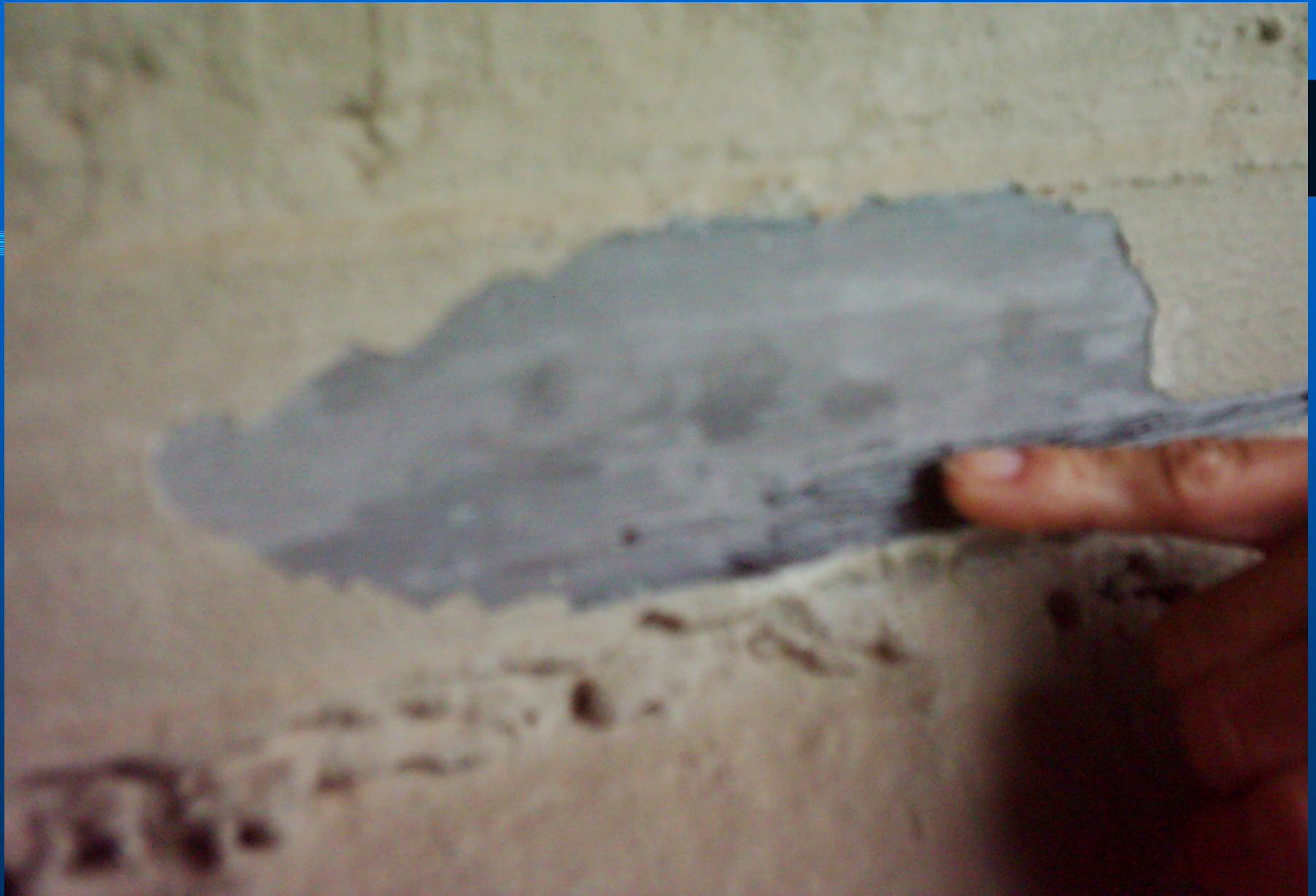
Picture 6: Some damages of protecting cover of FRP plates
