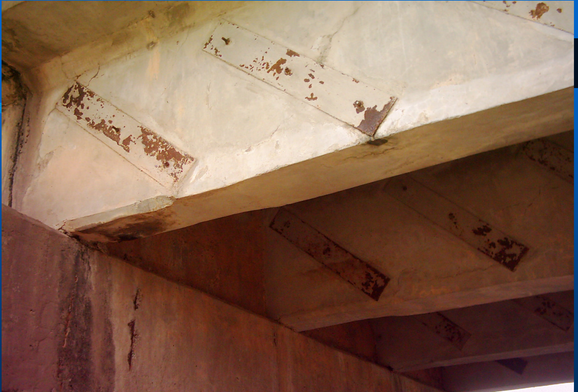
Picture 11: The rust in steel plate in wet place
