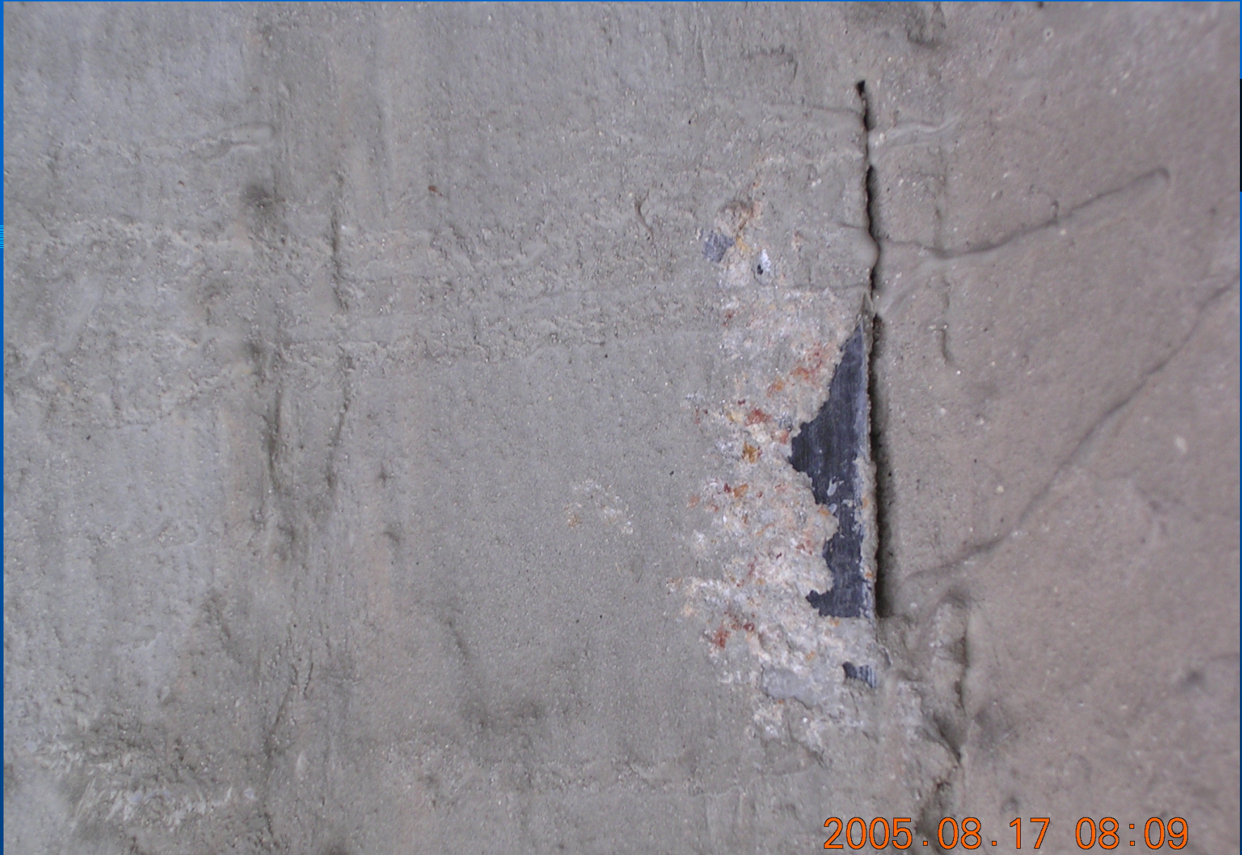
Picture7 : Some damages of protecting cover of FRP plates
