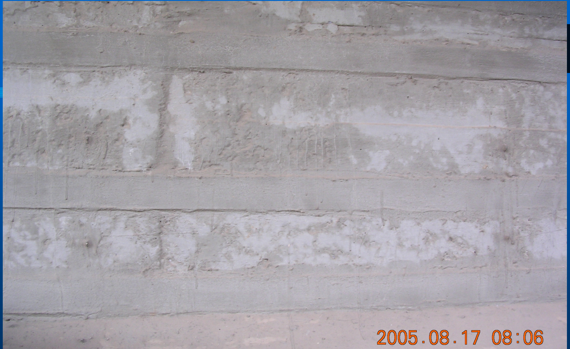
Picture 5: Location of protected FRP plates
