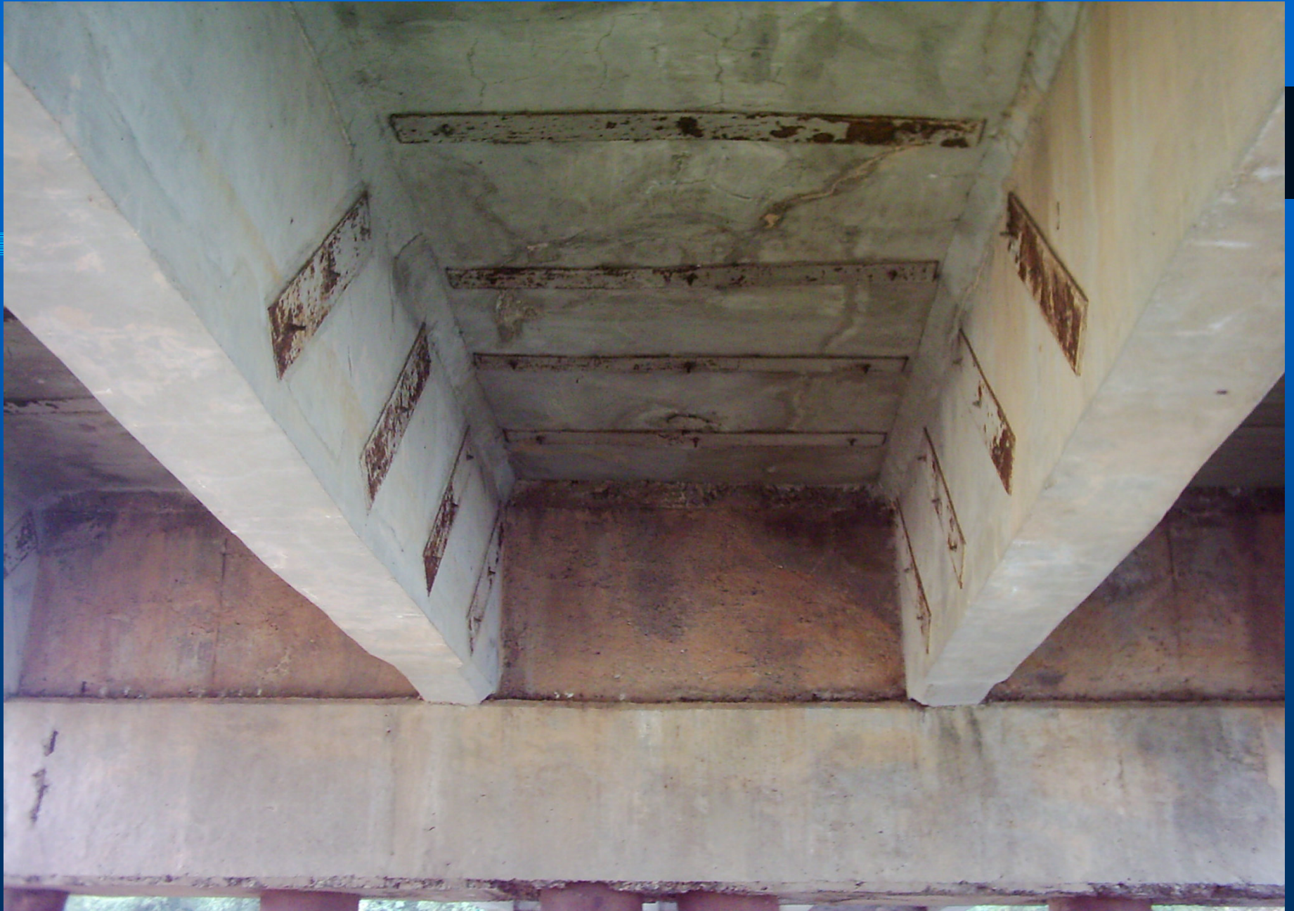
Picture 12: The rust in steel inclined plate in wet place
