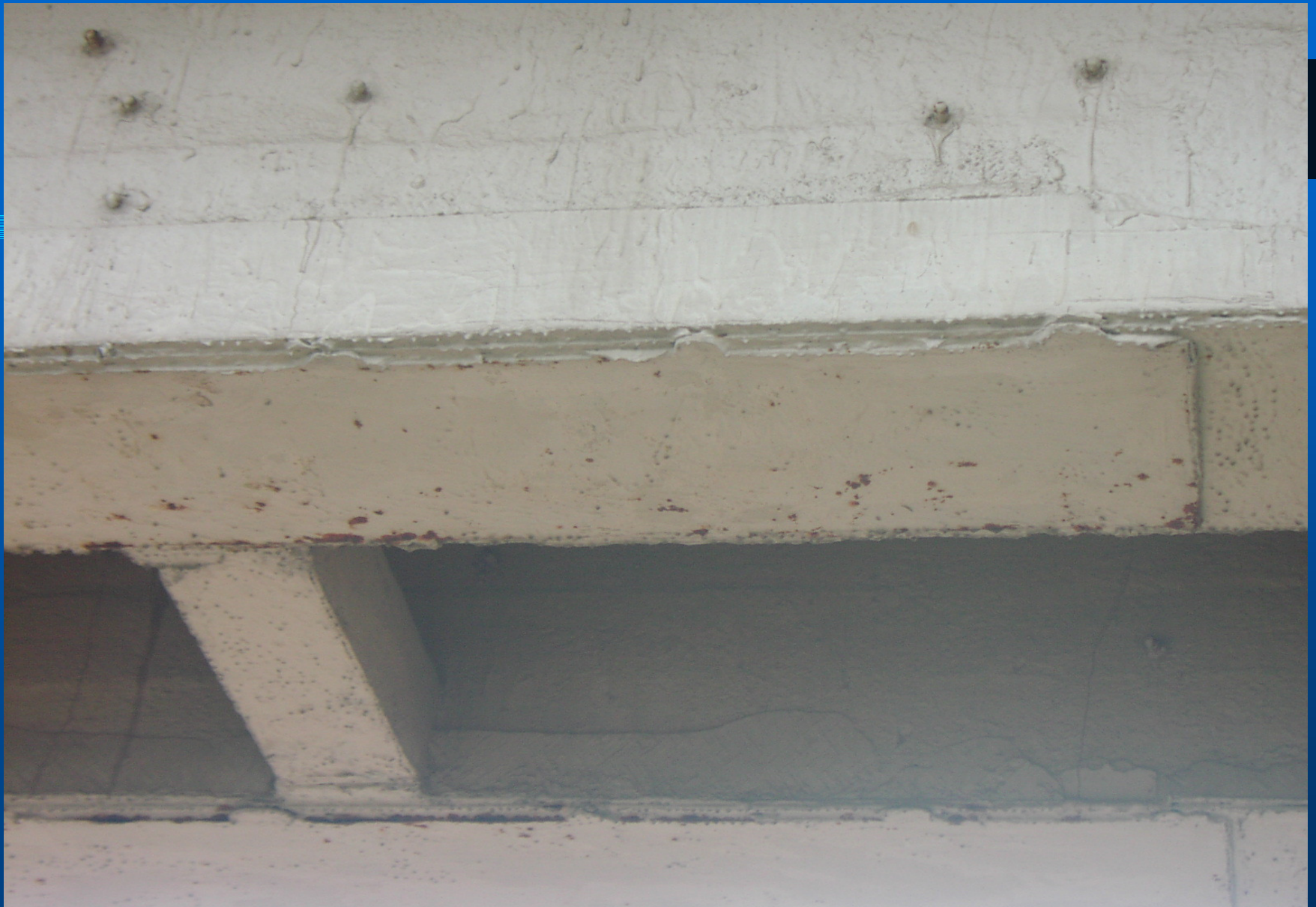
Picture 28: The steel plates after 10 years servicing
