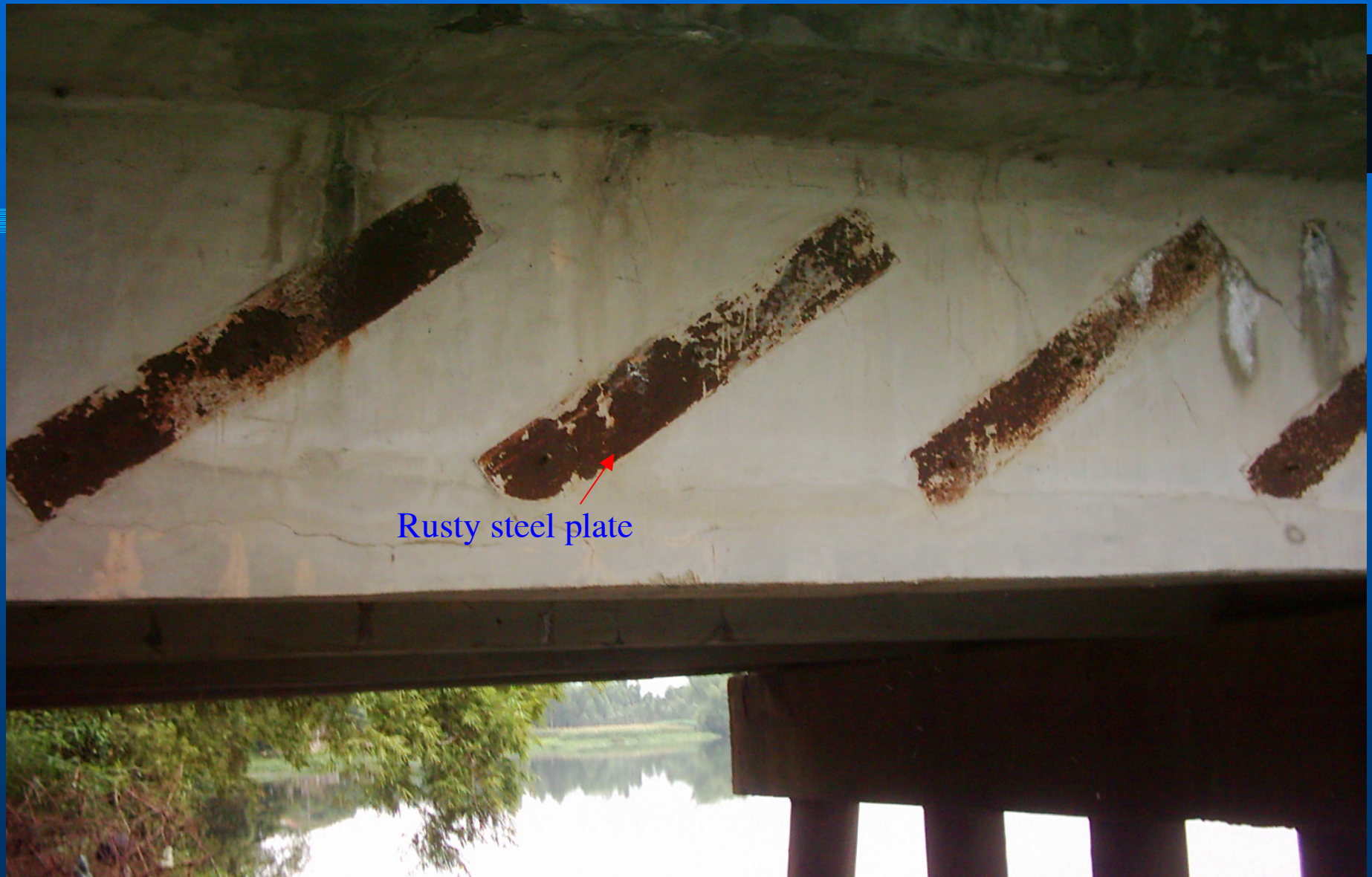
Picture 10: The rust in steel inclined plate in wet place
